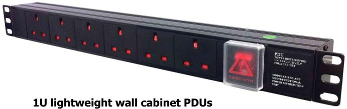
Picture shows 6 way horizontal UK 1U PDU
